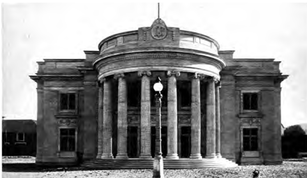
THE MISSISSIPPI BUILDING
