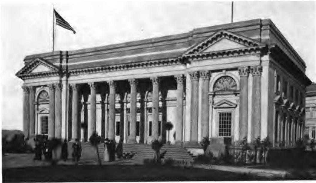
THE UTAH BUILDING
