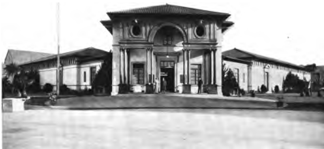
THE PHILIPPINES BUILDING
