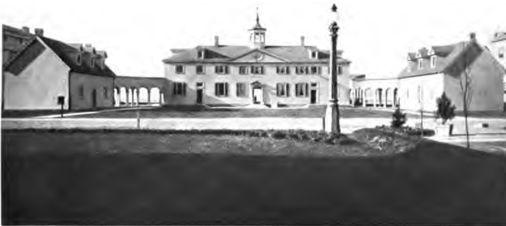
THE VIRGINIA BUILDING
