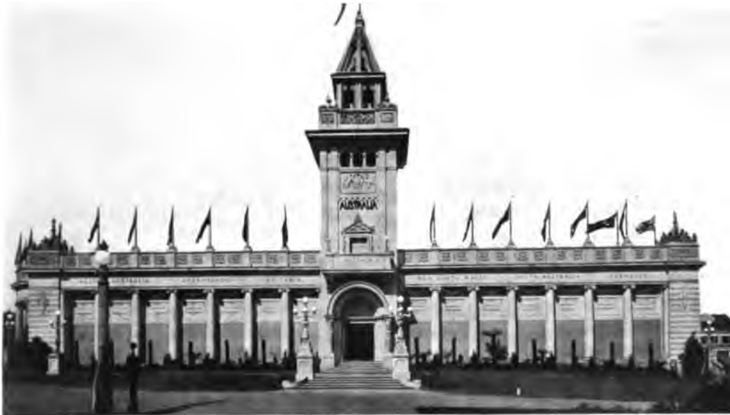
THE AUSTRALIAN PAVILION
