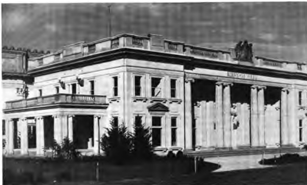
THE WISCONSIN BUILDING
