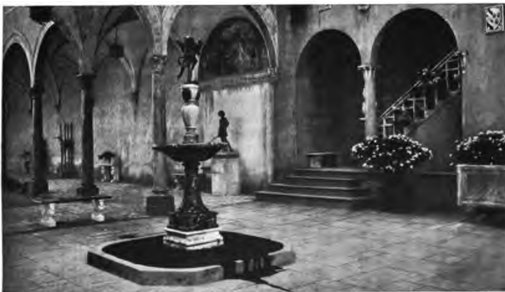
COURT OF THE ITALIAN PAVILION
