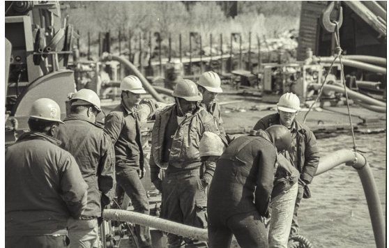
Harbor Clearance Unit TWO personnel at work on the barge deck during the clearance operation.
