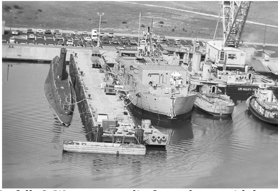
The Norfolk & Western wet slip from above, with barges, tugs and crane barge working the clearance. The scale of the obstruction that had to be removed before dredging could begin is plain.
