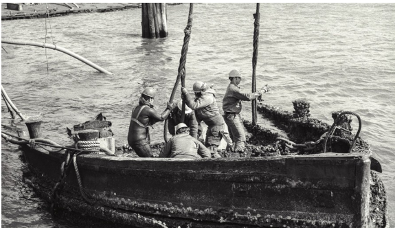
Hard-hatted salvage crew working from the gunwales of a small recovered craft awash alongside, hauling on a lifting strop. Old pilings stand in the background.
