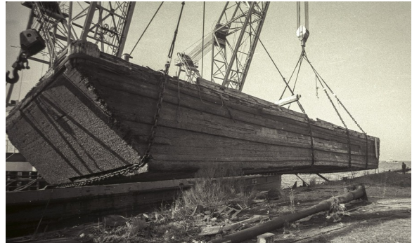
A long wooden lighter hull, its timbers thick with marine growth, hoisted stern-first from the slip and swung out over the debris field on the bank.
