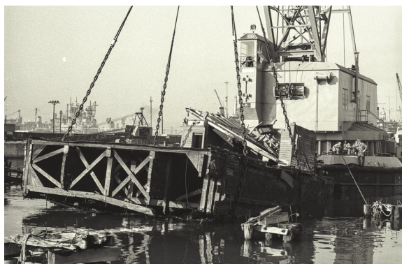
The crane barge lifting a heavy timber crib structure from the slip, a partially sunken vessel listing alongside.
