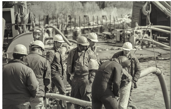
Harbor Clearance Unit TWO personnel on the barge deck during the clearance, hoses running past them to the work going on below.
