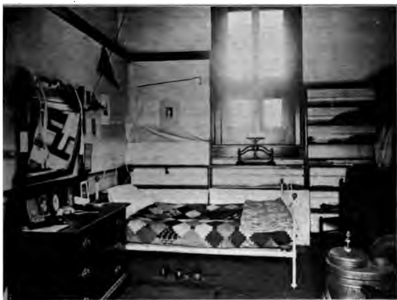
PRESENT INTERIOR, 46 EAST LAWN, UNIVERSITY OF VIRGINIA The "air-tight" has replaced the open fire of 1869
